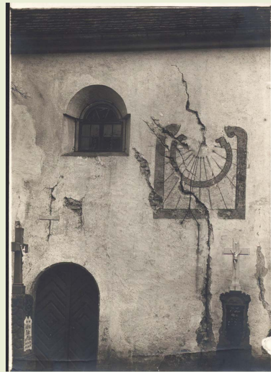
Figure 1: Earthquake damage at the church of Lautlingen due to 1911 Swabian Jura earthquake (LED archive, picture by FOTO BINDER, Ebingen).
